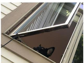
This picture shows wood rot on the bottom edge of the window. The builder did not seal or paint the outer window edges, leaving the frame exposed to moisture. This window is in dire need of repair or replacement (as noted by this inspector (a)).
