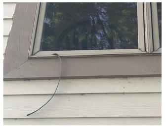
The above photo shows a seal that has become detached from the window. This seal is designed to keep moisture out of the wooden frame that encases the glass. If this seal separates, moister can enter the wood frame and hasten the rot. Owners may also have their glass frames sealed to offer an extra layer of protection against weather elements and prolong window frame life.
